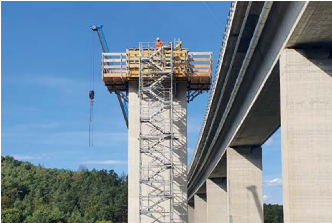
The imposing height of the bridge piers varies between 32 metres at the Auwiesenbach valley crossing and 56 metres at the Groisbach valley crossing, depending on the valley crossing.
