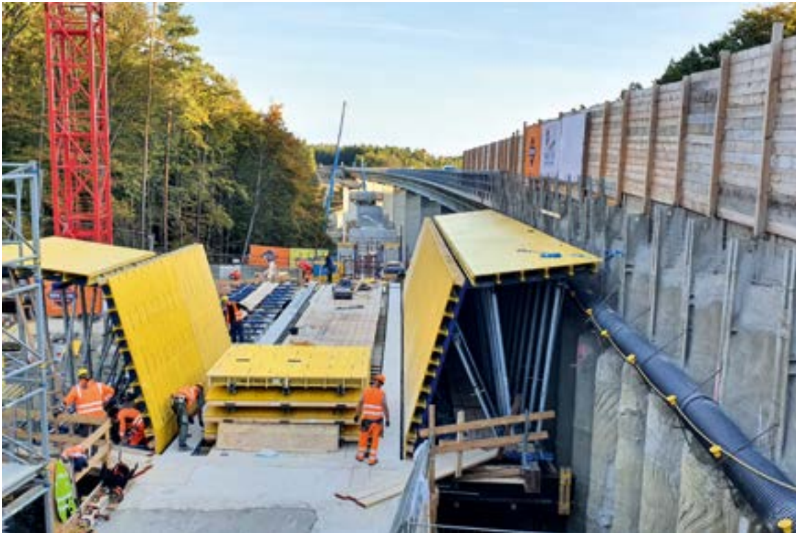
Three of the four bridges are being completed using the incremental launching method: The concrete elements are produced directly on the construction site and pushed in piece by piece using high-pressure hydraulic presses.
